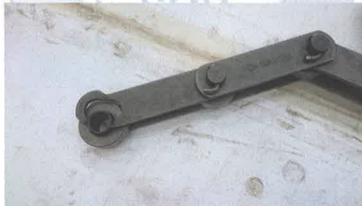
Photo. 3 – Mode of failure (ST628 - 70,000lbs)
